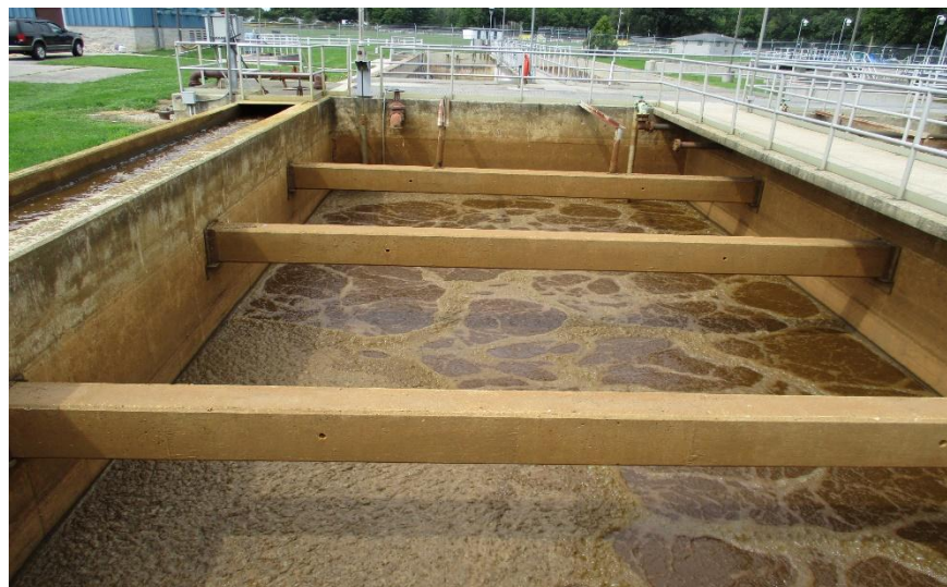
Figure 2-21 Aerobic Digester
