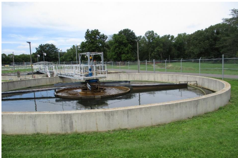
Figure 2-12 Circular Secondary Clarifer
