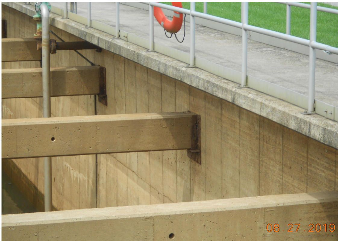
Figure 2-8 Concrete Support Beams in Aeration Tanks
